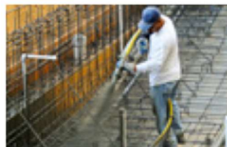
7 to 12 bar: Shotcrete applications
