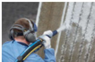
8.6 to 10 bar: Abrasive blasting
