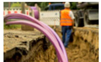
12 to 14 bar: Cable blowing and drilling
