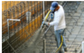
7 to 12 bar: Shotcrete applications
