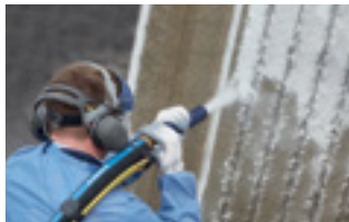
8.6 to 10 bar: Abrasive blasting
