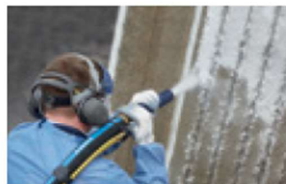
8.6 to 10 bar: Abrasive blasting
