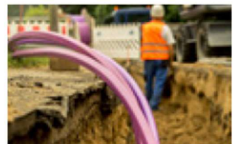
12 to 14 bar: Cable blowing and drilling
