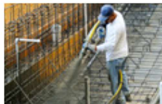
7 to 12 bar: Shotcrete applications
